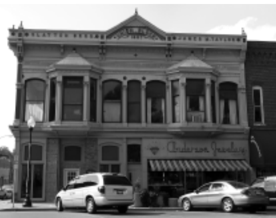
A “Mesker” storefront in Taylorville, Ill. Photo courtesy of Illinois Historic Preservation Agency.
